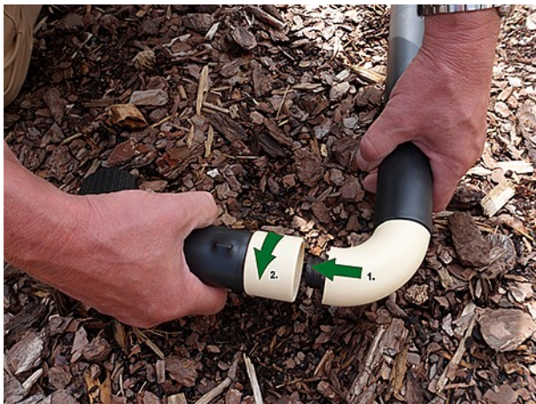
Illustration 4.14: Corner ready for assembly
